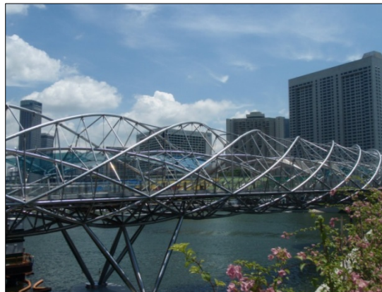
Helix Bridge, Singapur, 2011
